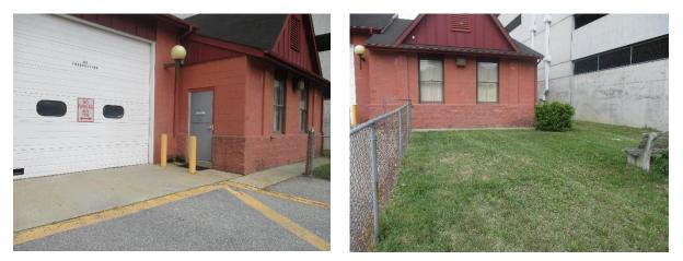
Pervious pavement can capture stormwater from the parking lot, and a cistern can capture stormwater from the roof of the building which can then be used for the needs of the fire company. A preliminary soil assessment suggests that the soils have suitable drainage characteristics for green infrastructure.
